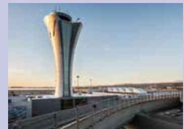
SFO Replacement Air Traffic Control Tower and Integrated Facilities
